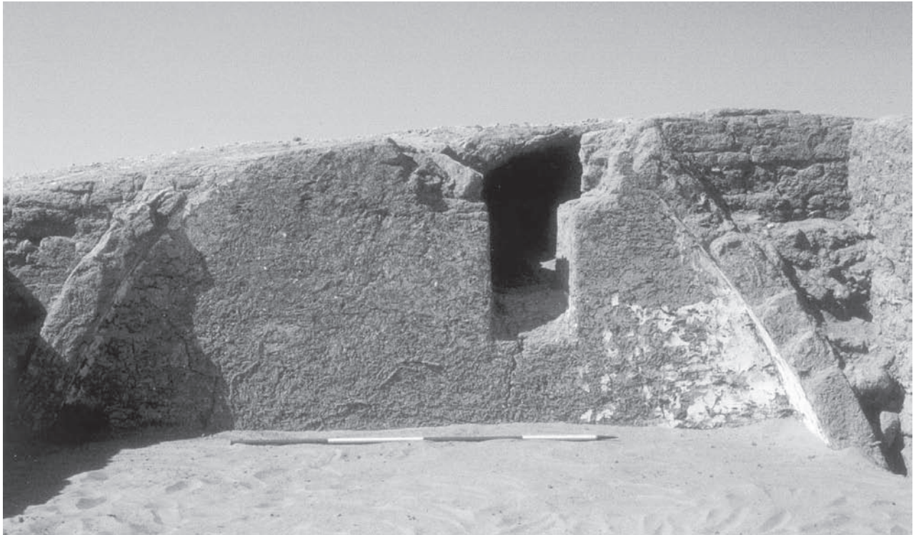
Plate 1 Small East Church, Room 2, west wall showing barrel vault and the window.
