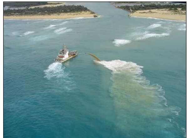
Figure 8. The April Hamer dredging at the offshore ebb-tidal delta during the ebb-tide. Source: Wheeler (2005)
