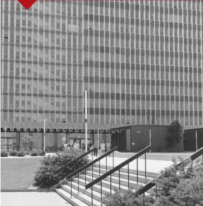
Menzies Building circa 1970 Image courtesy of Monash University Archive
